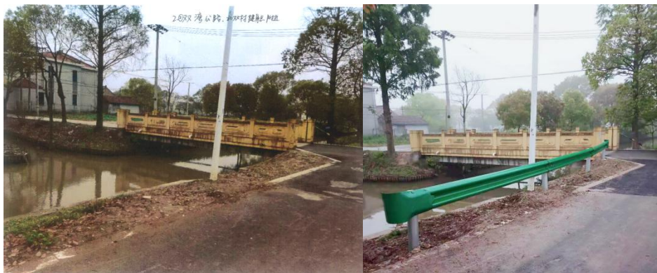
(临边护栏整治前后)
